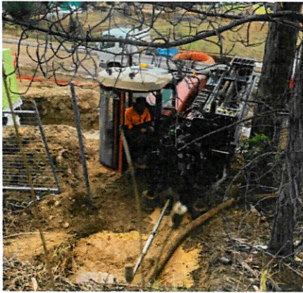
Typical Underboring Setup
